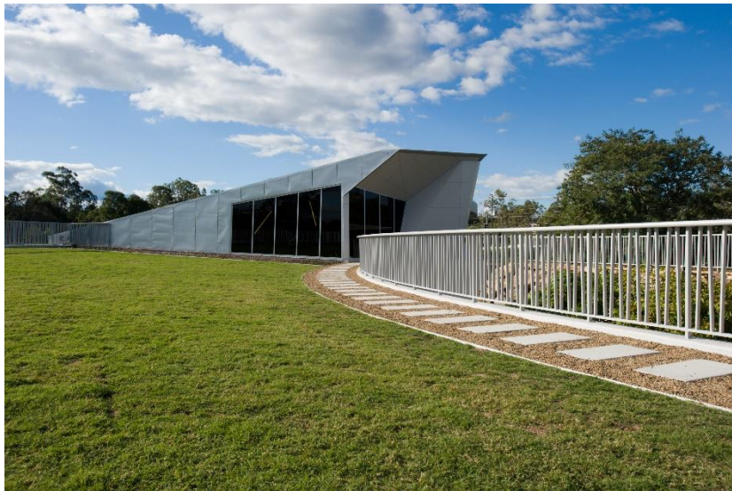
Figure 5. Cooroy Library grassy rooftop. Image credit: Phil Jackson courtesy of Noosa Library Services
